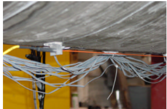
FIGURE 8. LONG GAGE LENGTH FIBER GRATING SENSOR MOUNTED ON THE BOTTOM OF THE BEAM
