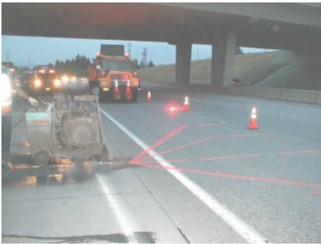
FIGURE 3. INSTALLATION OF FIBER GRATING SENSORS INTO THE I 84 FREEWAY
