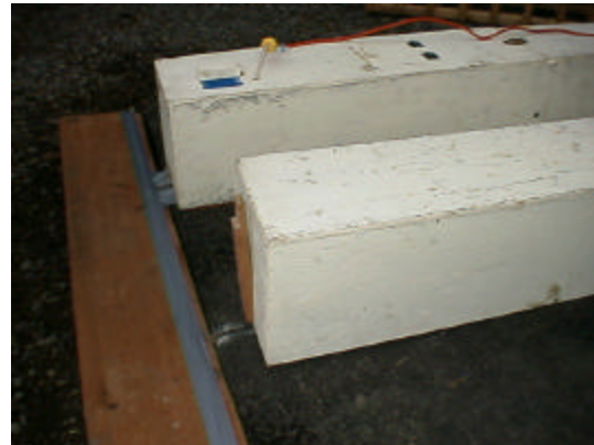
Figure 11. Heater boxes being used to cure epoxy.
