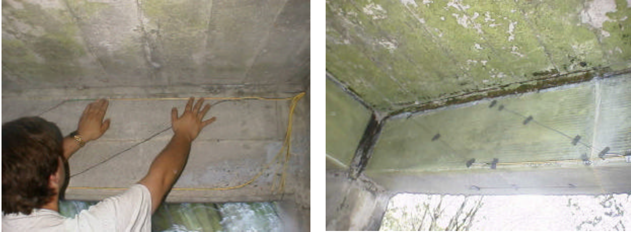
Fig. 6 Sensors being placed into grooves in the concrete (left) and embedded into the composite wrap (right)
