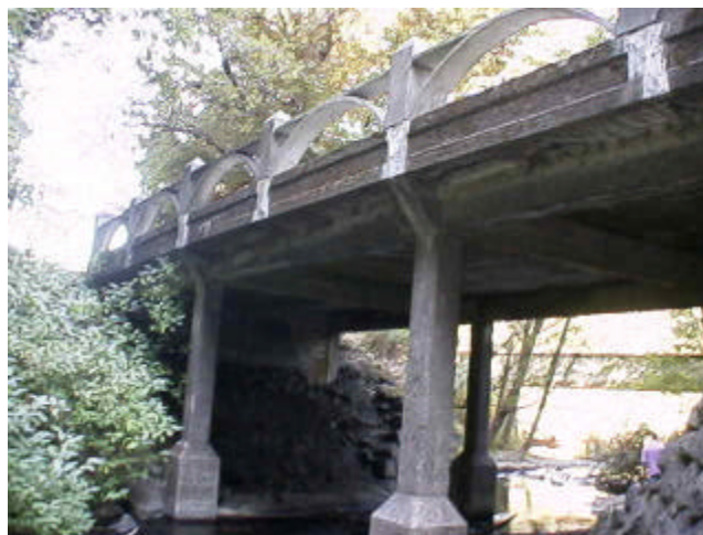
Fig. 5 Horsetail Falls Bridge before being strengthened by composite wrap and instrumented with 26 long gage fiber grating strain sensors
