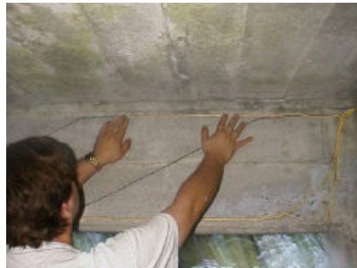
Figure 1. Horsetail Falls Bridge in the Columbia River Gorge National Scenic Area and 1.0 m fiber grating sensors used to support multipoint high speed dynamic strain measurements.
