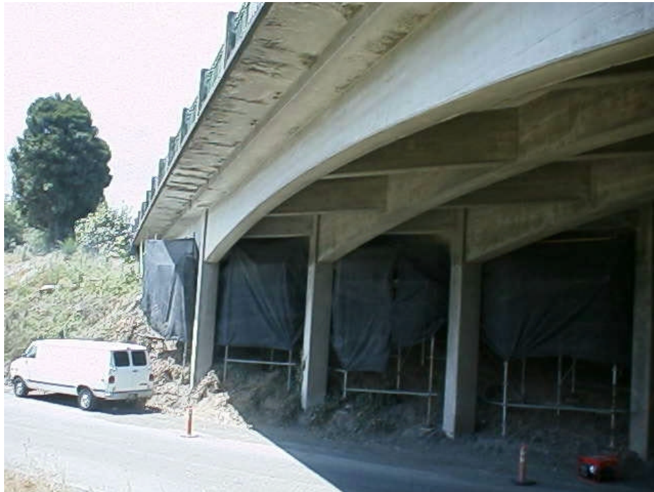
Fig. 8 Sylvan Bridge in Oregon scheduled for instrumentation mid July 2000
