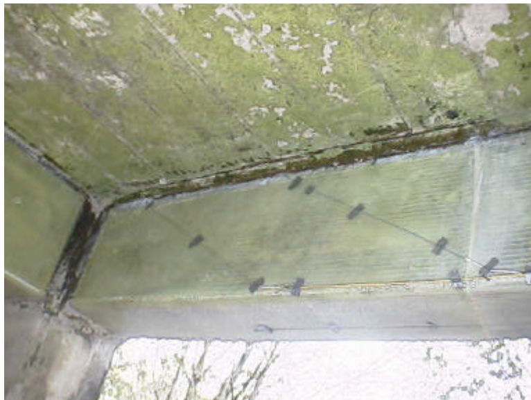
Figure 5: Sensors were mounted onto the glass-epoxy material after curing sufficiently.
