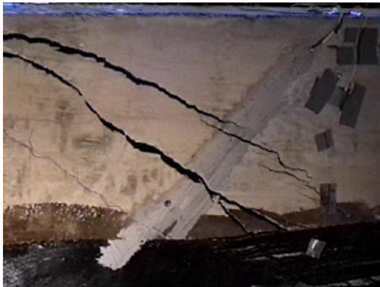
Figure 7: Shear failure in a full scale model concrete beam based on the Horsetail Falls Bridge beams.
