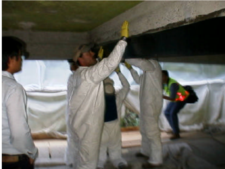
Figure 4: Installation of the Carbon-Epoxy Strengthening Material.
