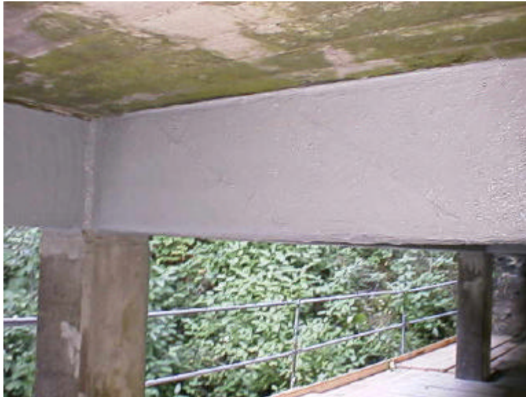
Figure 6: A cosmetic coat of epoxy was applied to the composites.
