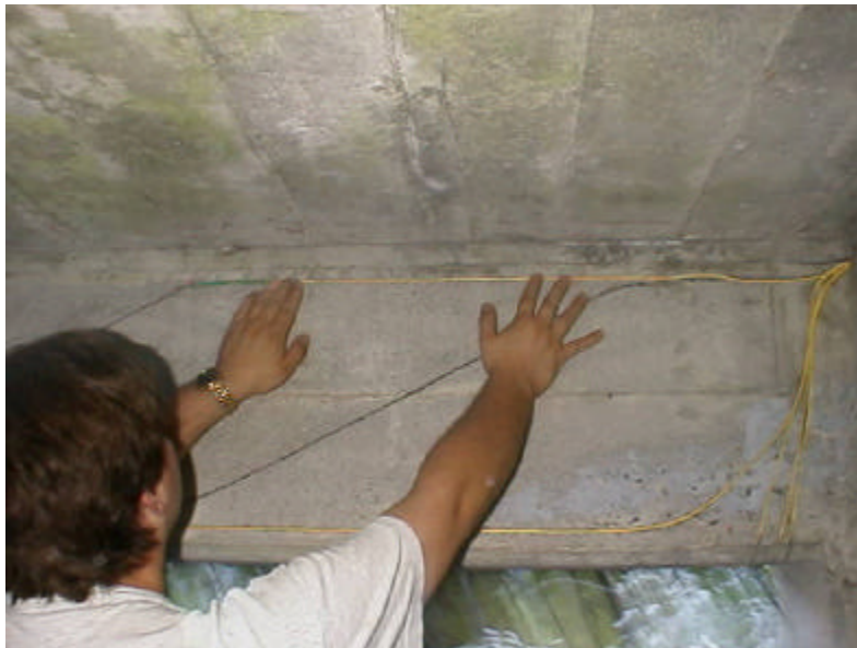
Figure 2: Installation of long gauge length bragg grating sensors into a beam.
