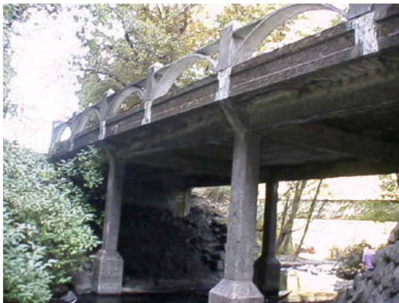
Figure 1: Horsetail Falls Bridge before the strengthening composite wrap was installed.
